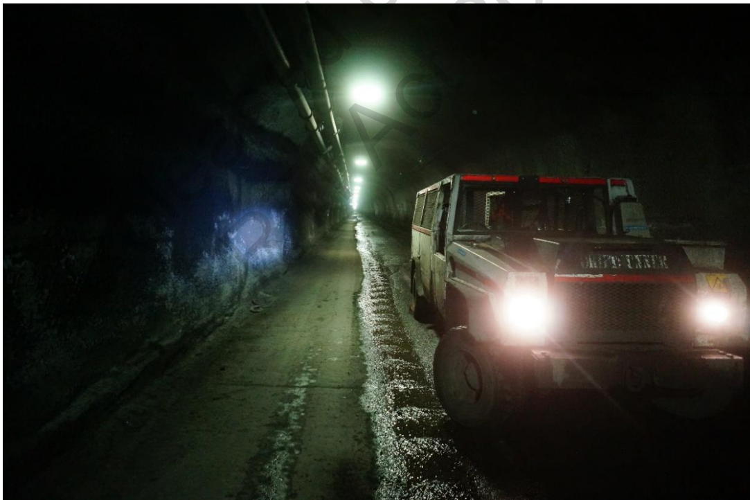
Figure 4: View down the drift from manhole 22 (A Driftrunner in the right foreground.)
