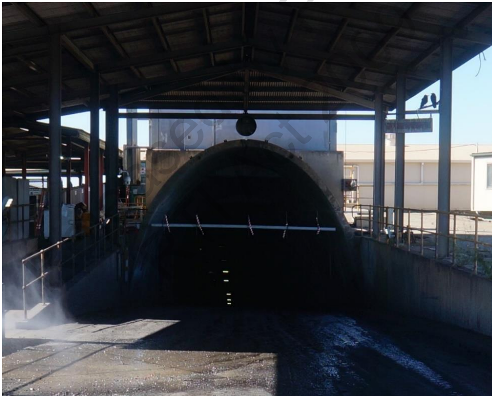
Figure 2: Moranbah North Mine Drift Entry
