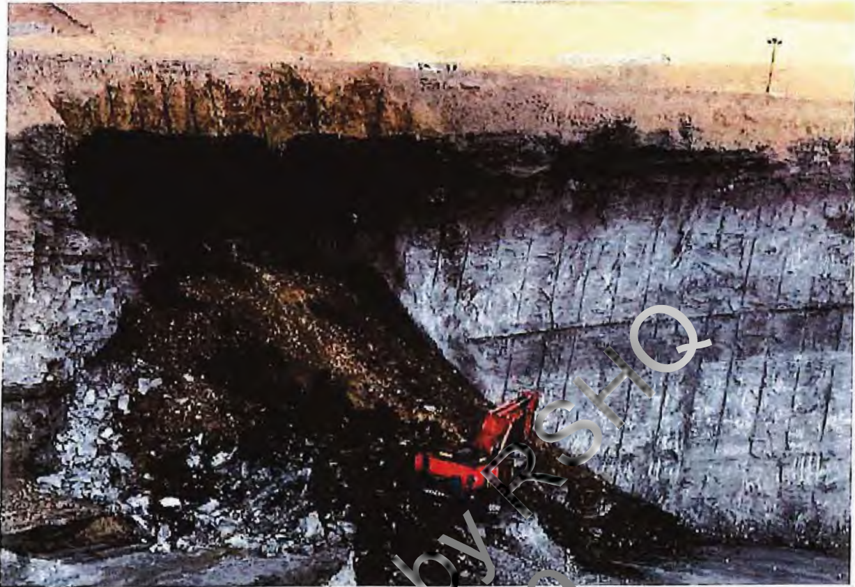
Figure 4. The failed pit wall that partially engulfed EX0046
