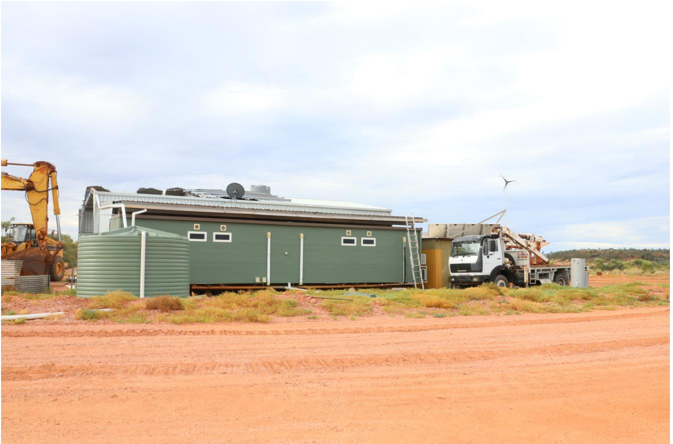
Photo 1: Workshop area layout – looking north (Note: Extension ladder used by Mr Selig to access workshop roof)
