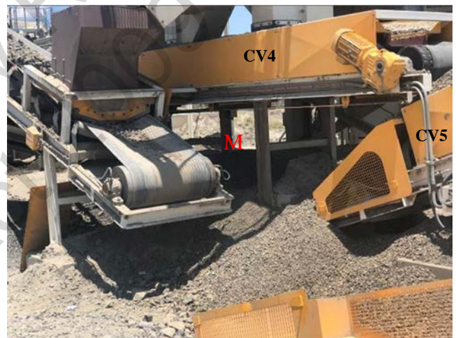
IMG_1269: Tail pulley of CV2. Rear guard is in foreground.
