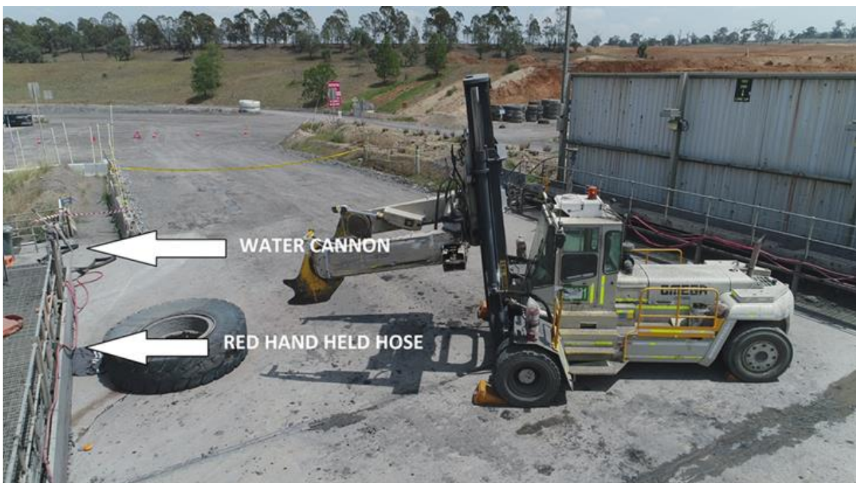
Figure 9 Heavy vehicle wash bay platform with water cannon and red handheld hose
